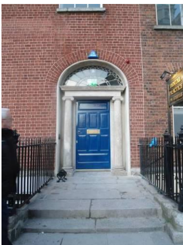
Rounded cutstone entrance with original fanlight and timber panelled entrance door
