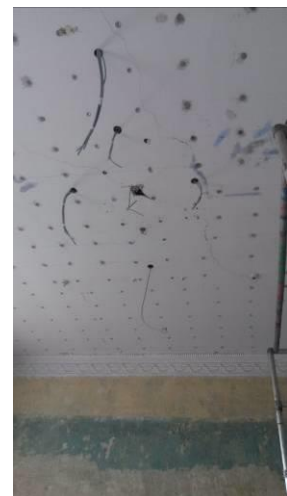
Ceiling consolidation using metal discs to support original ceiling
