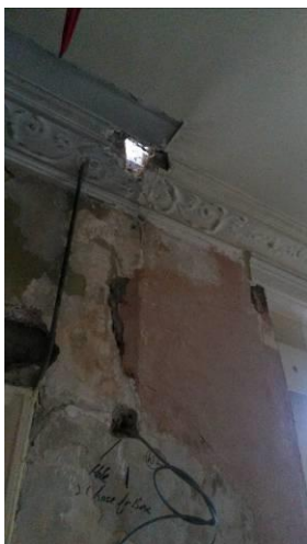
Damage to original cornices due to inappropriate building services integration
