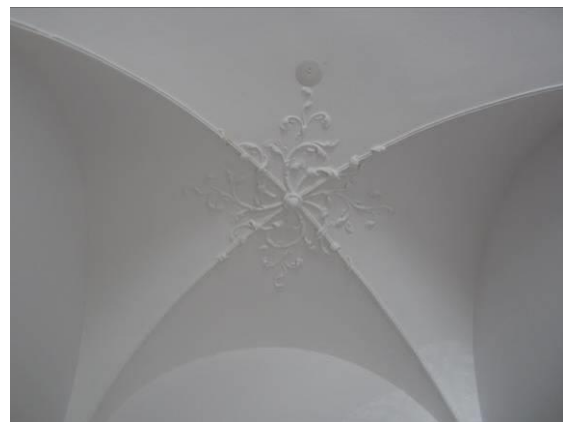
Original ceiling mould repaired with discrete building services
