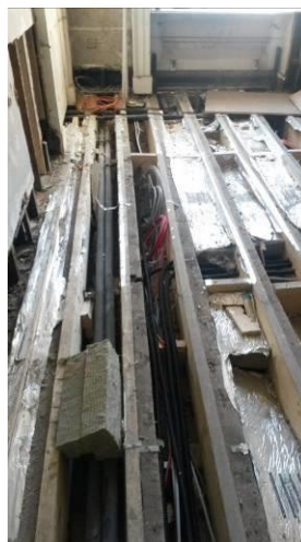
Pre-insulated multi-layer heating pipe-work between joists which were notched locally adjacent to radiators
