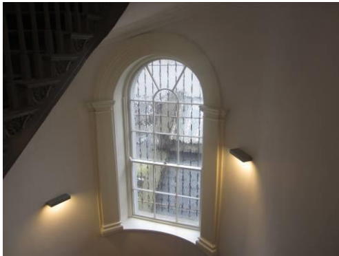
Refurbished window; rich-grey painted stair treads enhance architectural detailing
