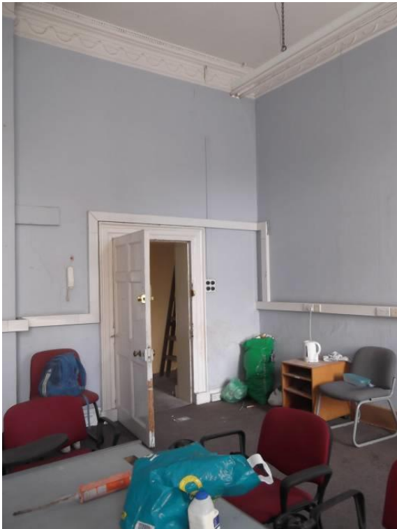
First floor seminar room prior to refurbishment
