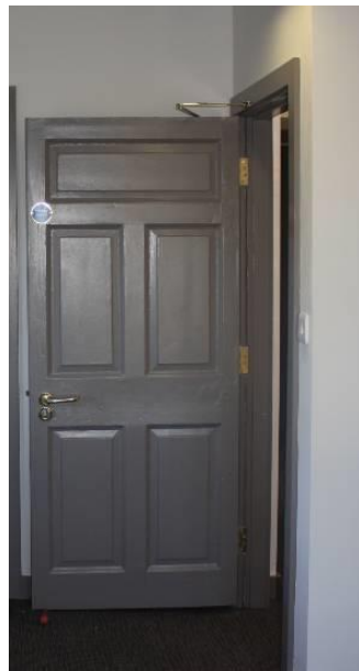
Existing door upgraded with hardwood slips and intumescent strips and coating
