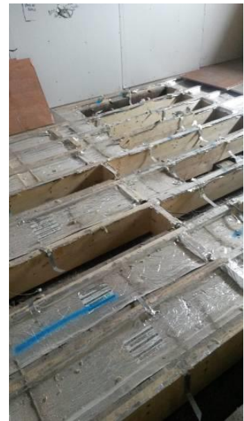
Rockwool Flexi between existing floor joists
