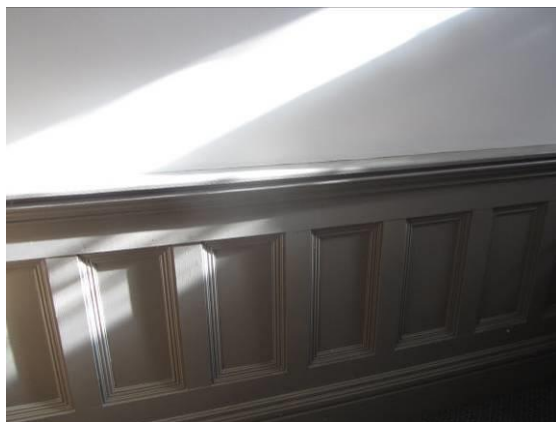
New wainscoting to entrance hall
