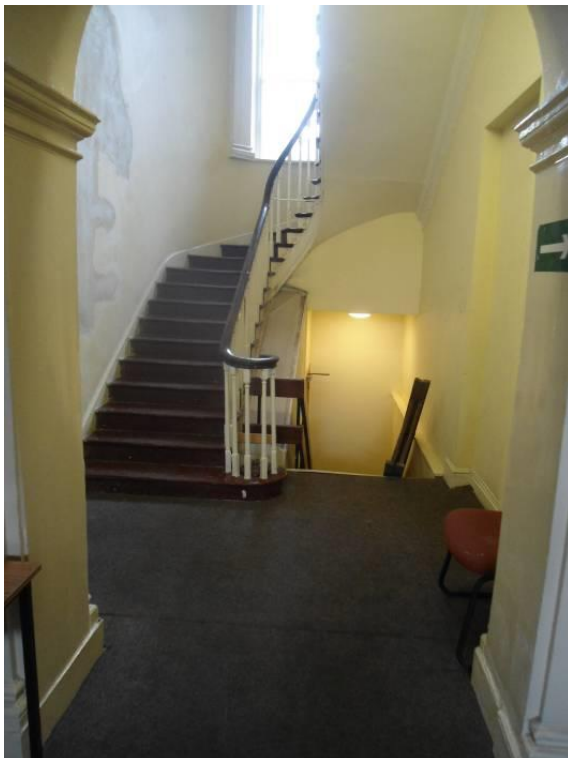
Curved stairwell prior to refurbishment
