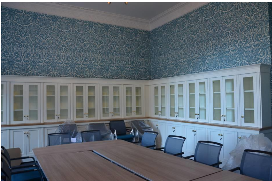
Built-in shelving incorporating state of the art audio-visual equipment, with hand-crafted wallpaper finish and repaired cornice to seminar room
