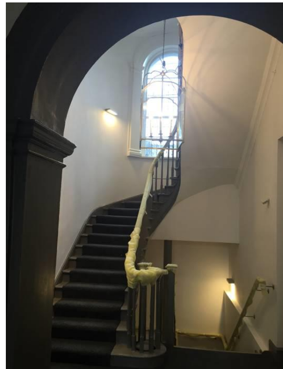
Curved stairwell after refurbishment works completed
