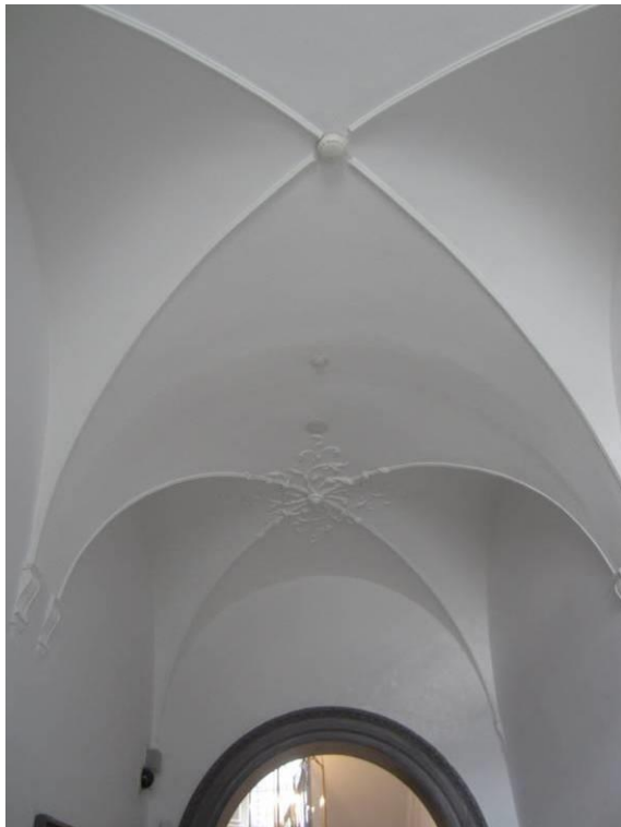
Original ornate moulded ceiling to entrance hallway
