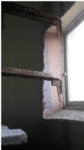
Glass fibre mesh used within Eco-mortar R100 lime plaster to internal walls
