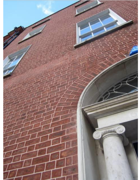
Tuck pointint carried out to red brick walls during first phase of works.
