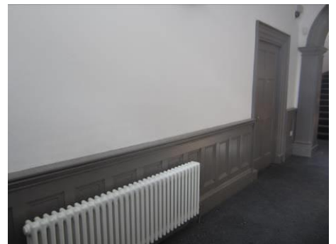
Traditional appearance radiators help retain the domestic Georgian character of the building
